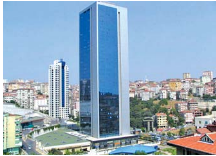
Polat Towers Residence, İstanbul
