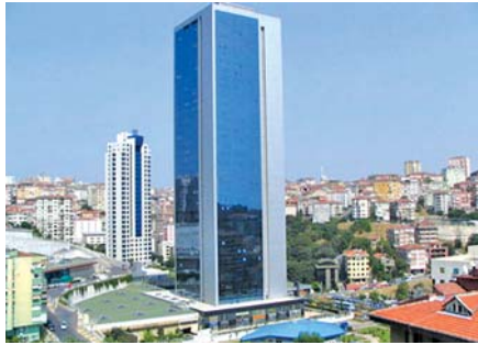
Polat Towers Residence, İstanbul
